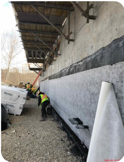
Perimeter waterproofing
