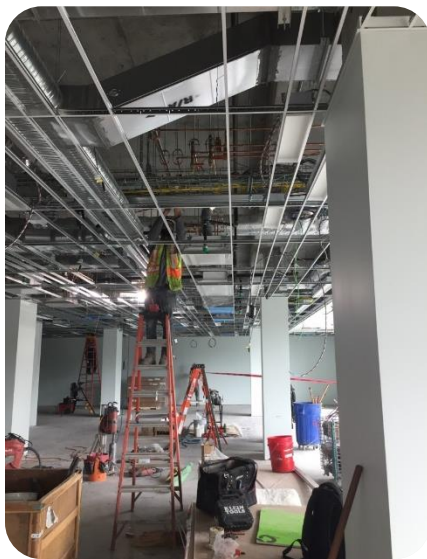
Walk-in clinic ceiling grid
