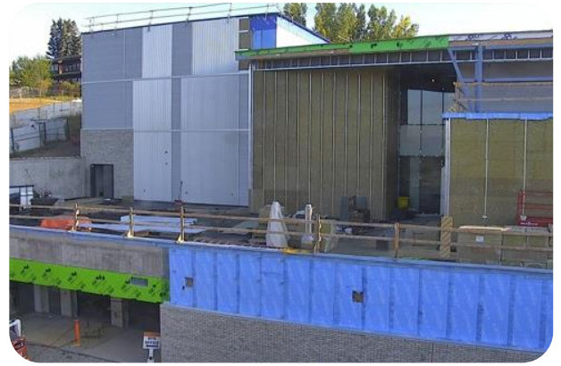
2nd floor rooftop garden – exterior cladding
