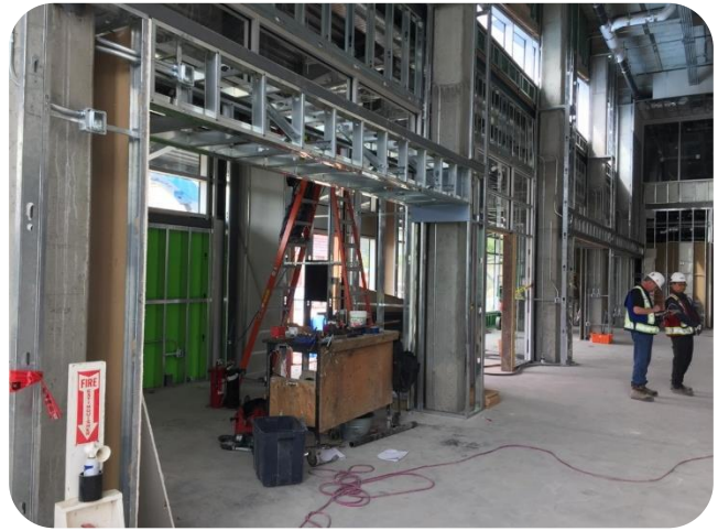
Main floor south rooms framing
