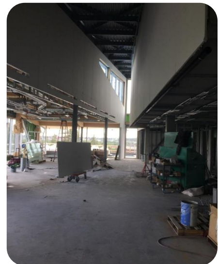
Day Hospital lounge bulkheads
